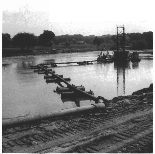
Monument with pontoons: The Pumping Derrick. (Photo: Robert Smithson.)
